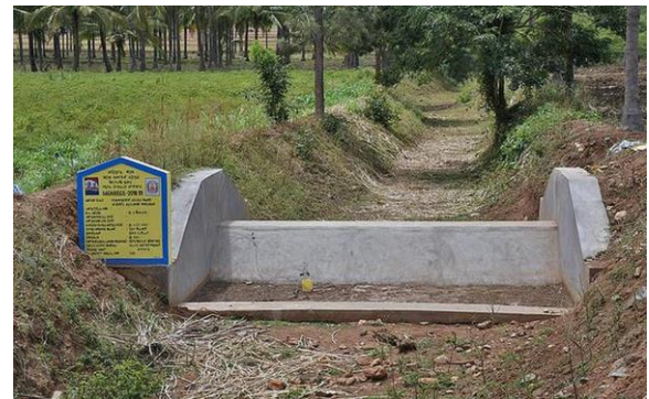
Figure-6.2. Construction of a Check Dam
